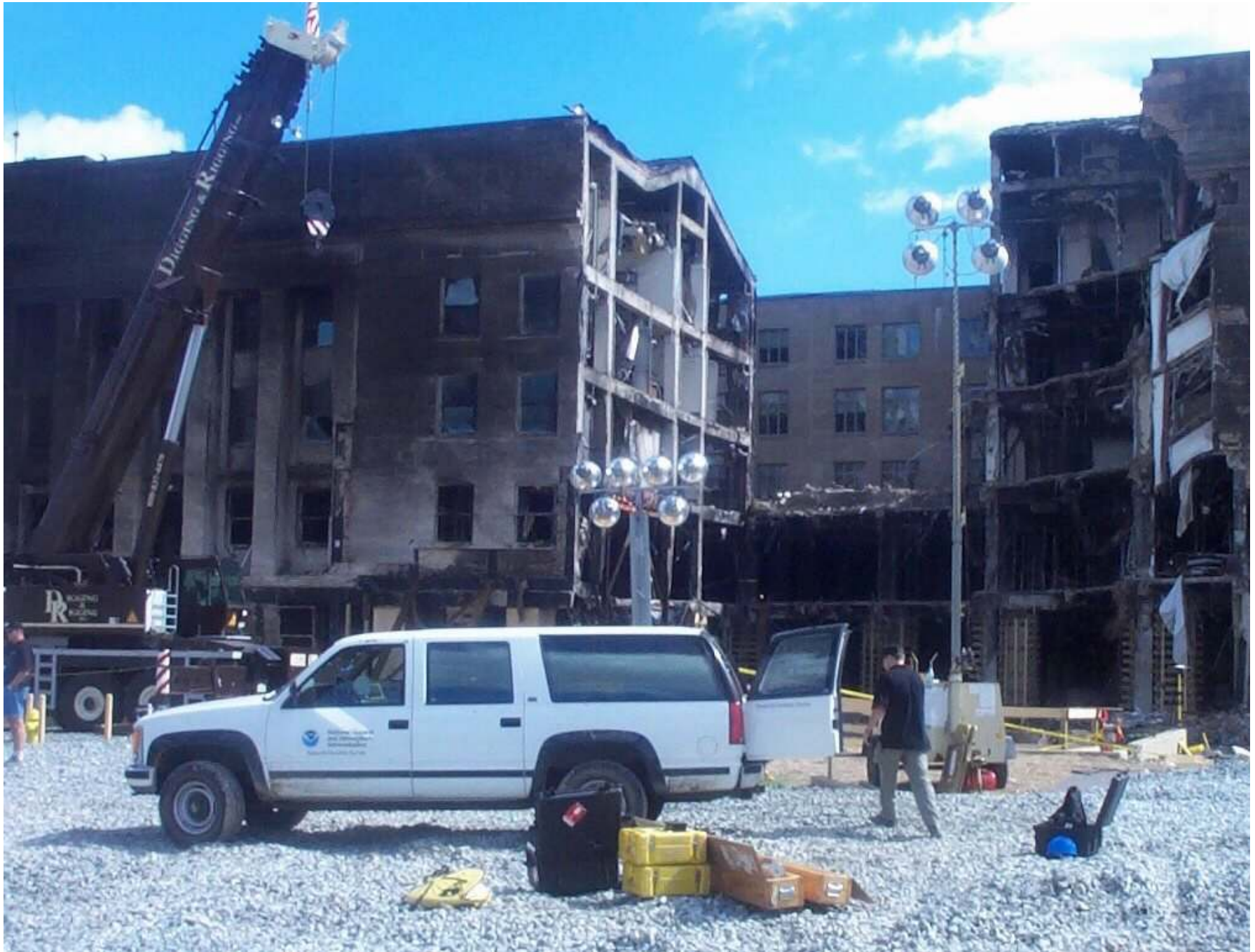
NOAA Truck and equipment being set up at Pentagon
